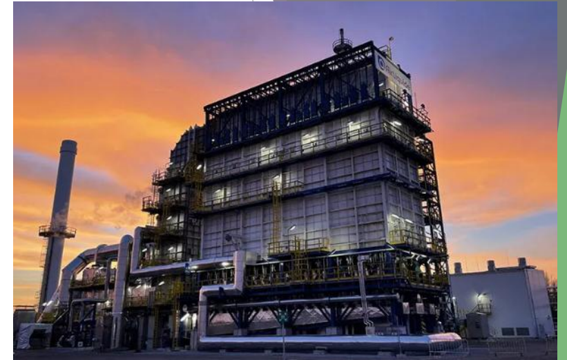
Air Liquide SMR plant in Anwerpen (B)
