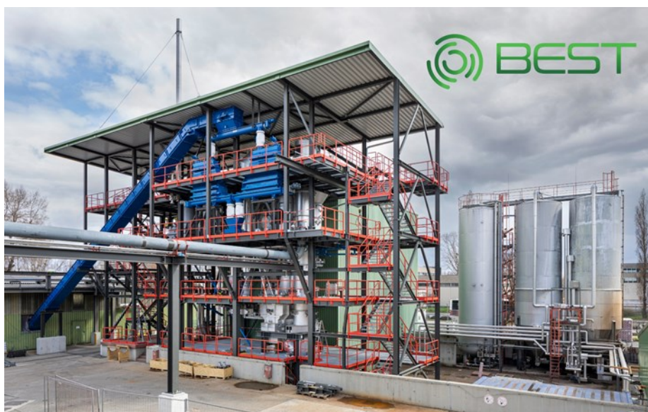
Figure 3: The 1 MW DFB steam gasification demonstration plant at the Syngas Platform Vienna
